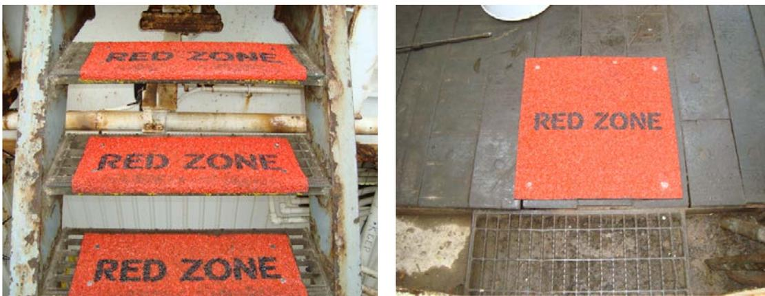
**Figure 3 Example Red Zone Marking Techniques**
